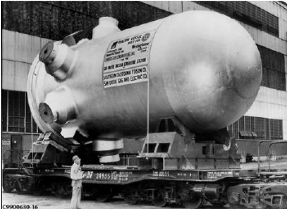
▶ Vessels may weigh up to 800t with wall thickness up to ~330mm.
